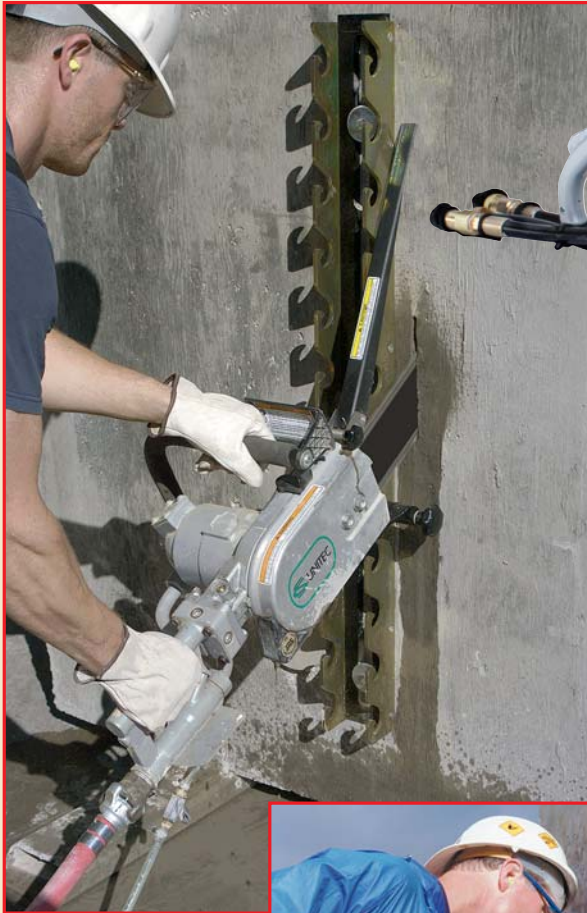
Above: Optional SpeedHook® guides saw for straight cutting (see page 26).
