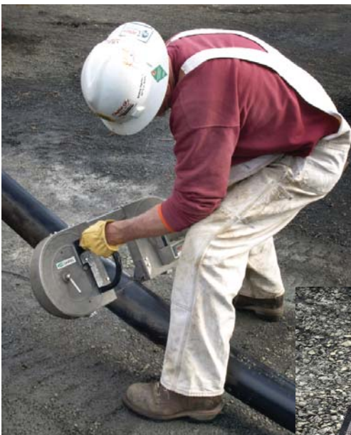
Above: New River crew member cuts high-voltage transmission cable.
