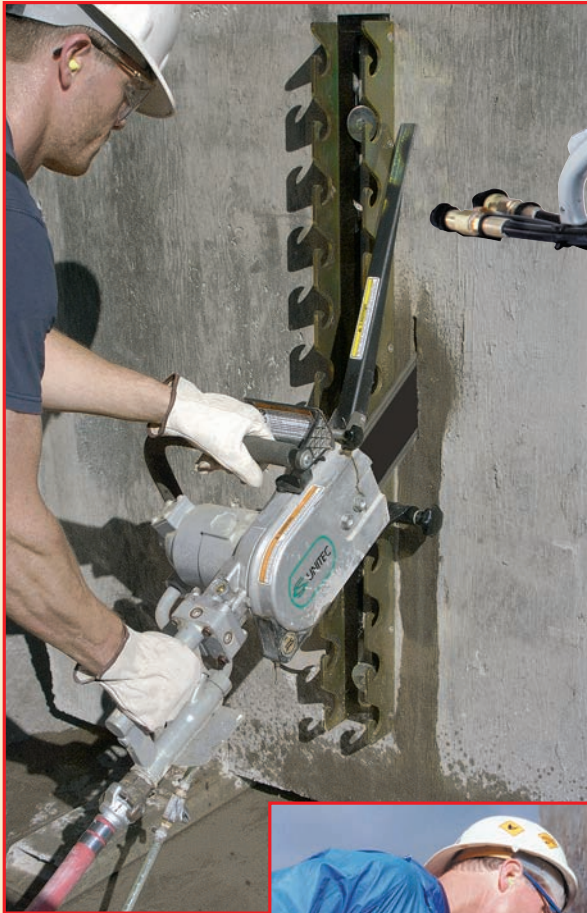
Above: Optional SpeedHook® guides saw for straight cutting (see page 30).
