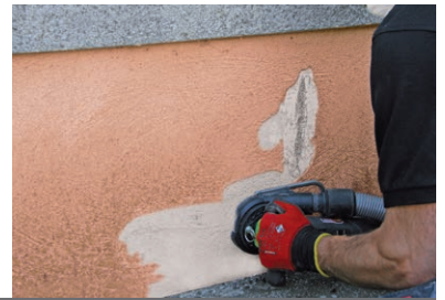
PCD milling disc for concrete surfaces (P/N 37125)
