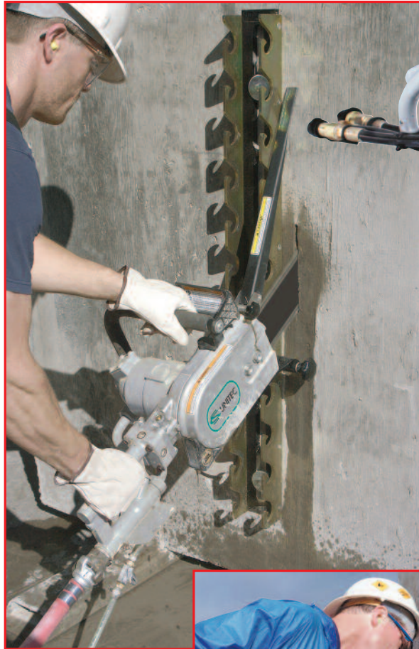
Above: Optional SpeedHook® guides saw for straight cutting (see page 34).
