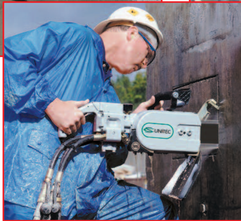
Above: Optional SpeedHook® guides saw for straight cutting (see page 34).
