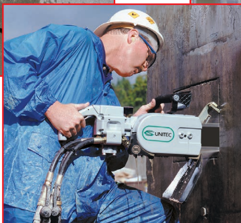
Above: Optional SpeedHook® guides saw for straight cutting (see page 36).
